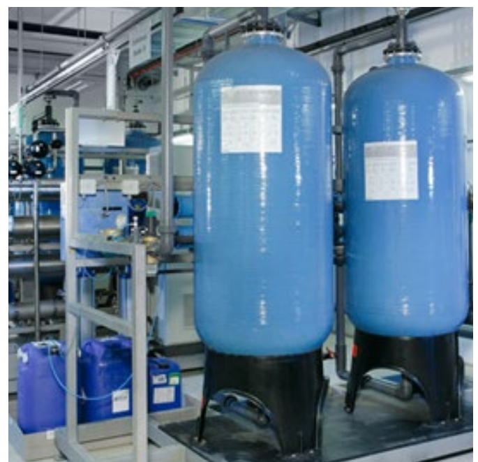
Ion exchange for process water preparation (e.g. boiler feed water)
