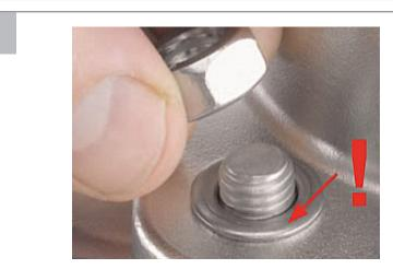
• Position the connecting bolts from the body side and bolt together diagonally with the valve body/nuts so that they are hand tight (do not use force).
